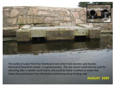
erosion. The invert of the two culverts is about 1.5-2 ft above high water (tide). Back in 1984 ACT suggested removal of boards for the winter- that remains a good recommendation. A drop structure and streambed protected against erosion on the discharge side should be considered. The Association may wish to contact DEP-Fisheries to determine whether there is interest in re-establishing anadromous alewife passage since the elevation and proximity to the Sound is close.
